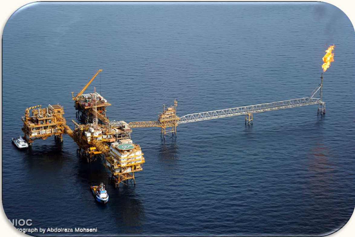
Abouzar production platform, the largest Iranian oil production complex in the Gulf. Photo courtesy of National Iranian Oil Co.
