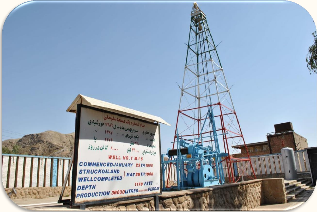
Above: the first successful oil well in Iran, Masjed Soleiman-1
