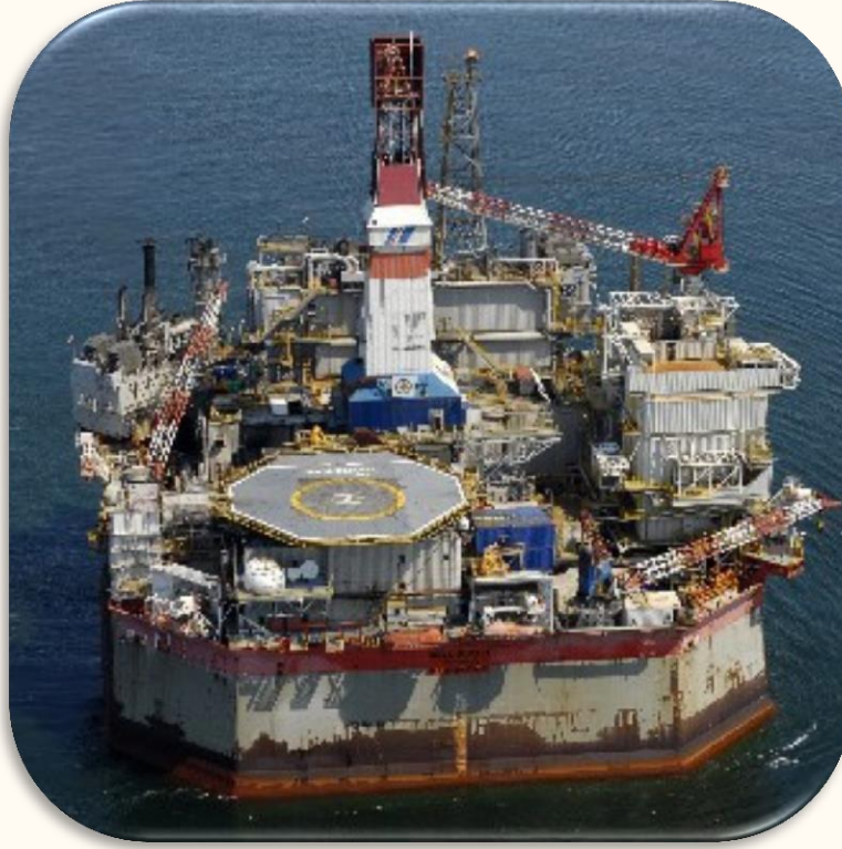
Above: The first oil platform installed off the Arctic coast of Russia Photo courtesy of Rigzone
