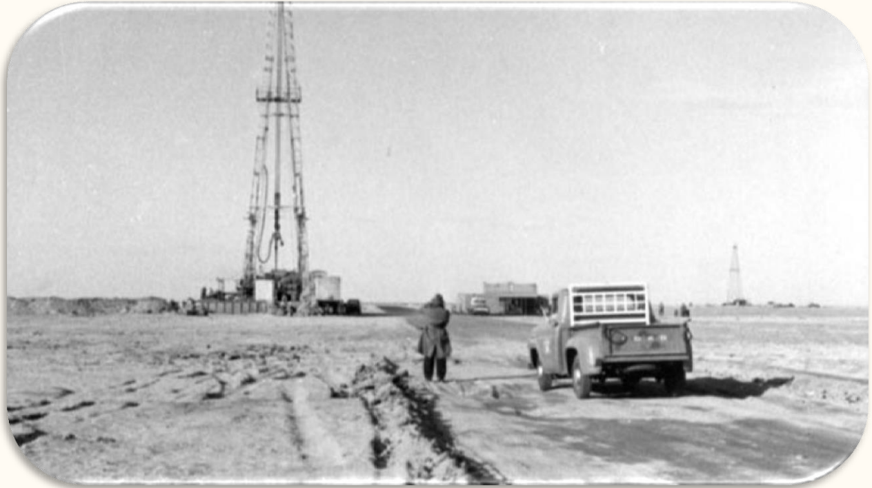
Drilling activities in Sinai, Egypt. (1970s). Photo courtesy of Eni.
